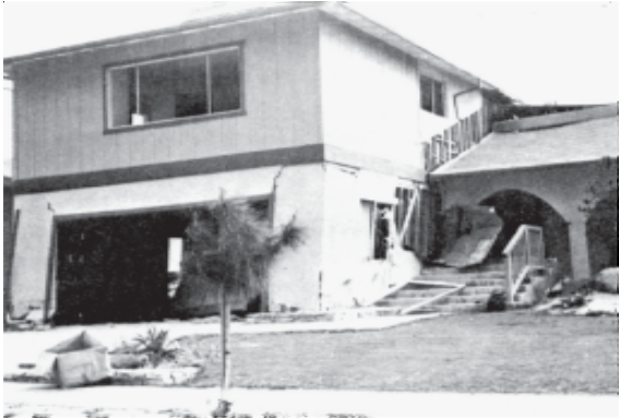
Figure 1 - San Fernando Earthquake, Feb. 9, 1971 Severely damaged split level 1 and 2 story wood frame dwelling. The one story portion dropped about 3 feet.
