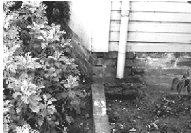
Figure 20 - Note the bricks exposed in this unreinforced masonry foundation.
