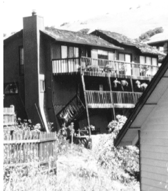
Figure 22 - This hillside home was built on an unbraced tall wall that failed.
